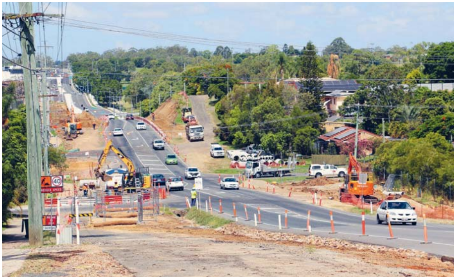
The next stage of the Redbank Plains Road upgrade has started
