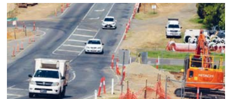
Stage two work at Redbank Plains will cost $7.6 million
