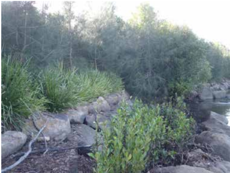
12-1-12: LWD & rock structure stabilised bank, plants established
