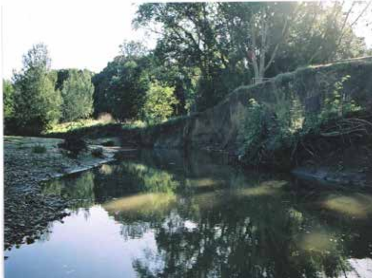
Currumbin Creek: Pre-restoration Extreme erosion, scouring, slumping, bank loss
