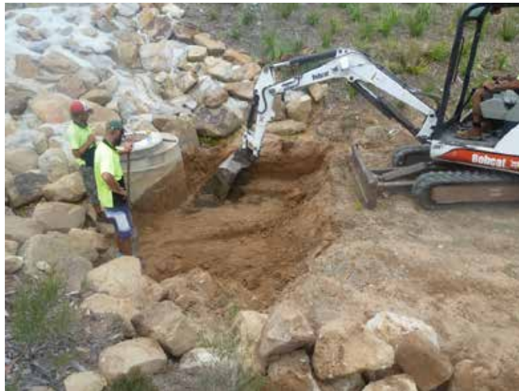
Springfield Lakes Estate, Ipswich: Plunge Pool construction
