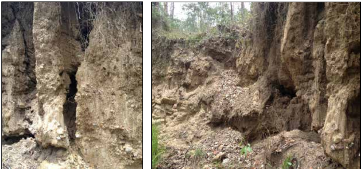
Figure 6-1 Expression of tunnelling on exposed creek banks within Zone 1b
