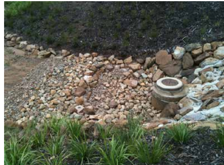
Springfield Lakes Estate, Ipswich: Rock Chute construction
