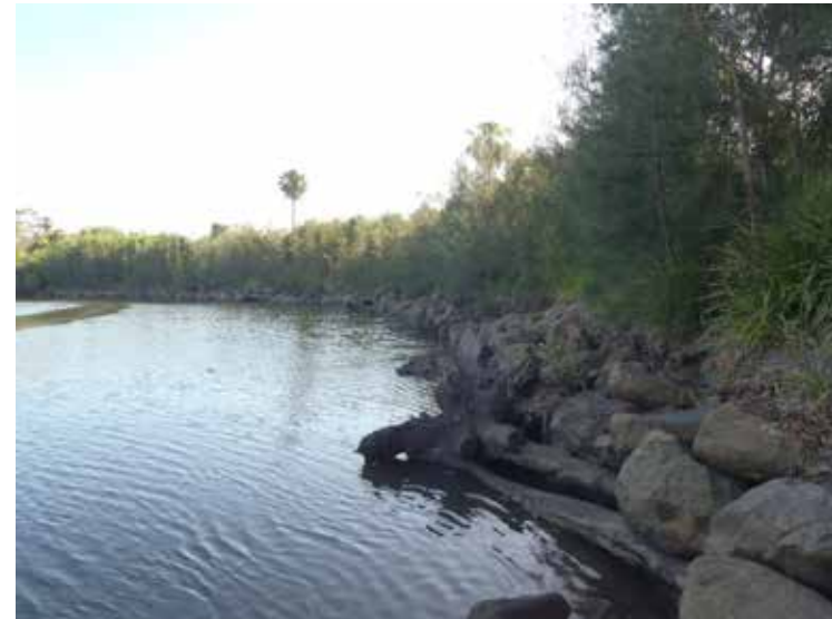
12-1-12: bank erosion halted. Riparian reveg established
