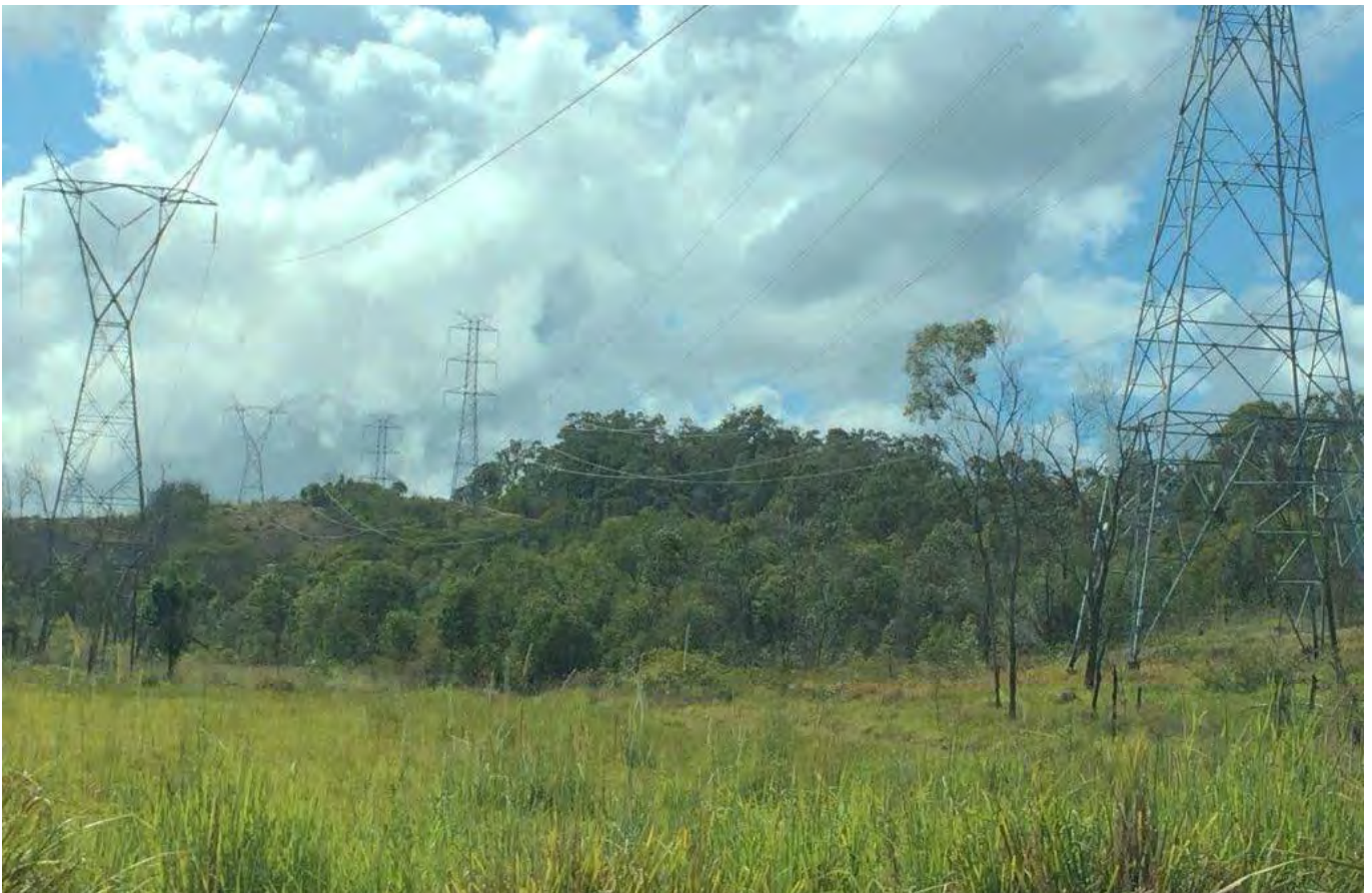
View along part of the high voltage transmission line in the estate
